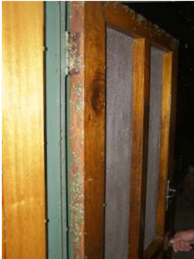
Rate of entry through a closed screen door. Note top edge as well.
